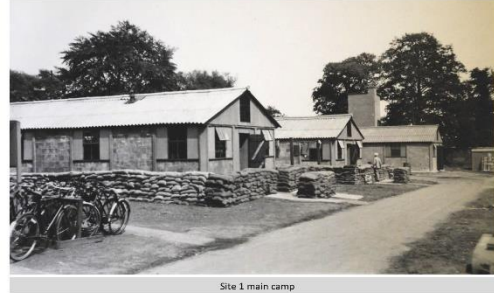
Site 1 main camp
